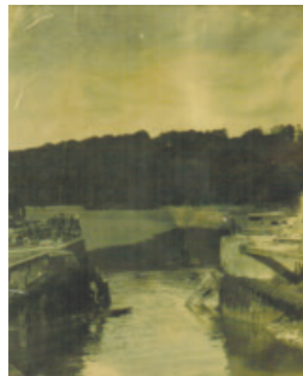
Remains of swing bridge at Dunkettle House after being blown up by anti-Treaty Forces Sept 1922
